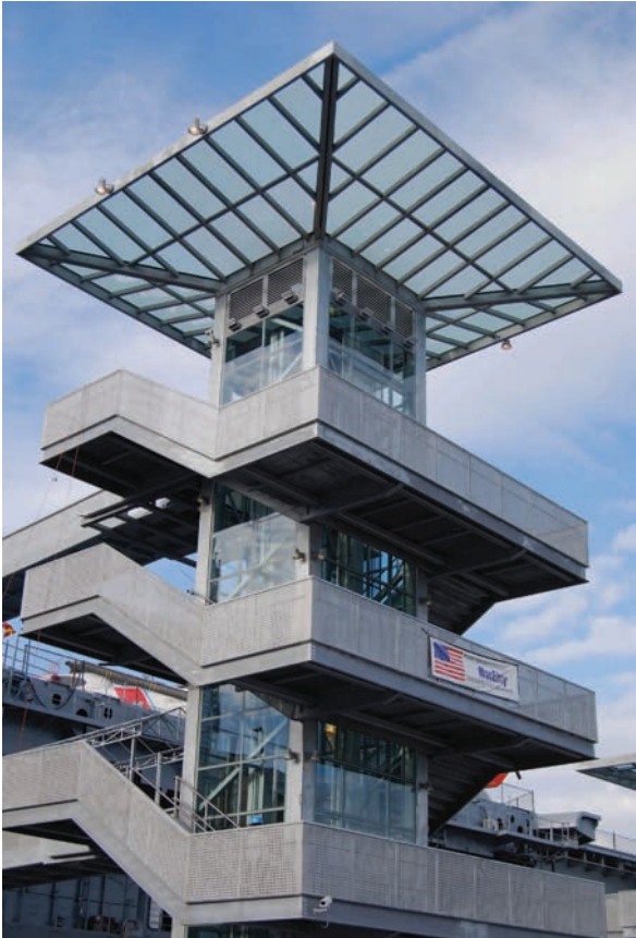
USS Intrepid Gangway Infills New York Dattner Architects
