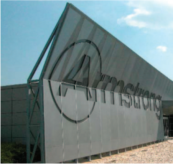
Perforated Sign for Armstrong Visitor Center Lancaster, PA Audrey Matlock Architect
